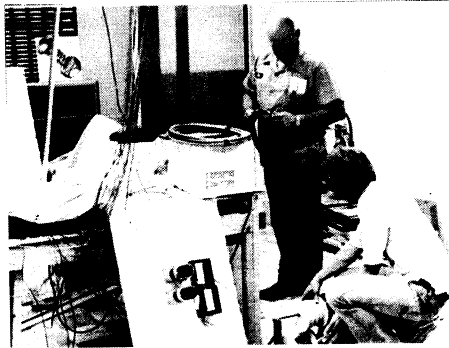
Work in Progress: WNDR is presently undergoing renovations to make room for an additional studio.
