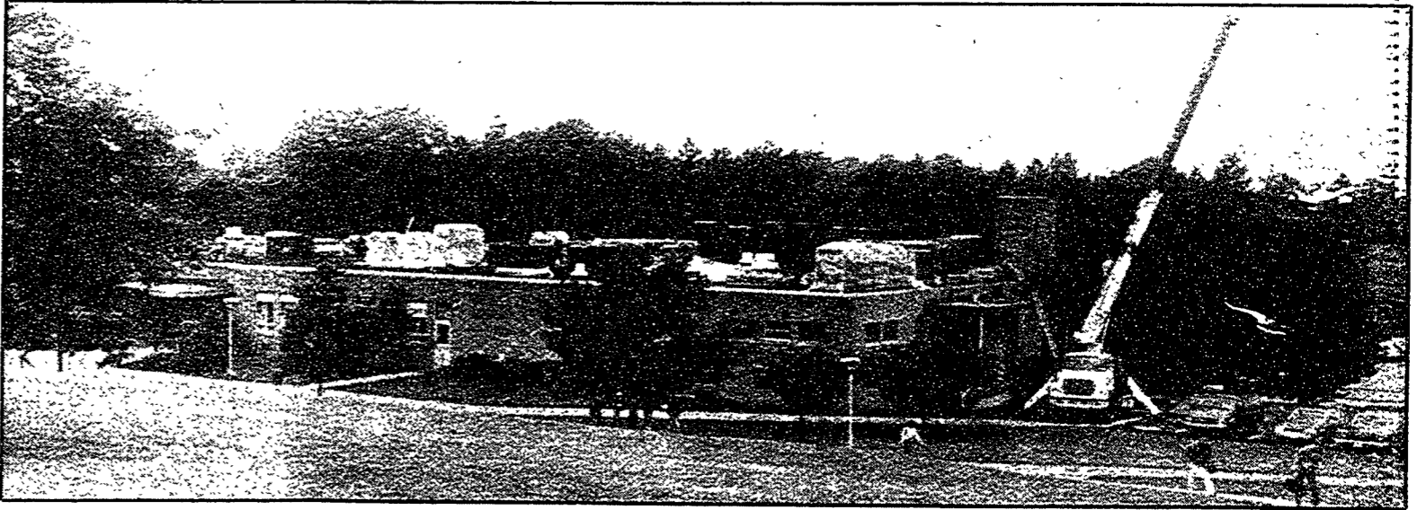
The Reed building gets a new roof.
