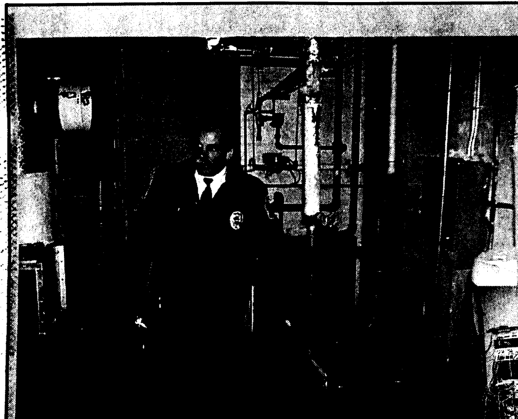
Officer Robert Truitt points out the septic system that was one of the problems during the floods in the fall semester.
