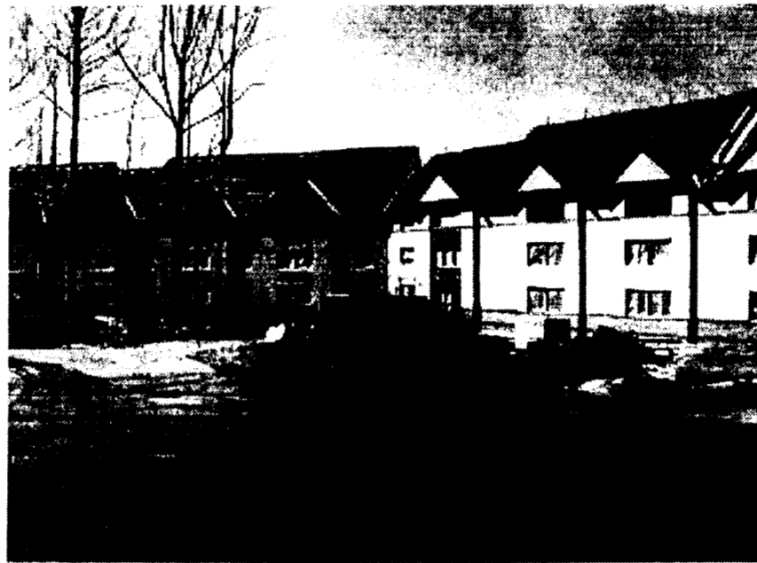
Ohio Hall under construction
